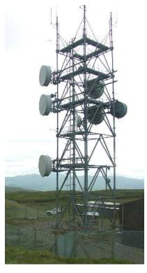
Figure 6a. Microwave repeater showing multiple co-located antennas.[3]
